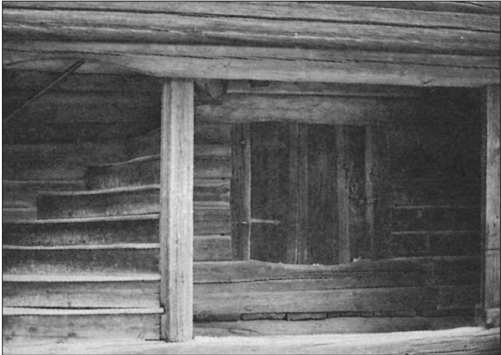
Figure 14.3: Solid, untreated timber has very good moisture-regulating properties.
