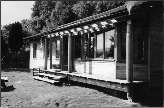
Figure 19.1: Nettleton Cabin in central Scotland, constructed from locally-sourced, untreated timber. Source: Howard Liddell
