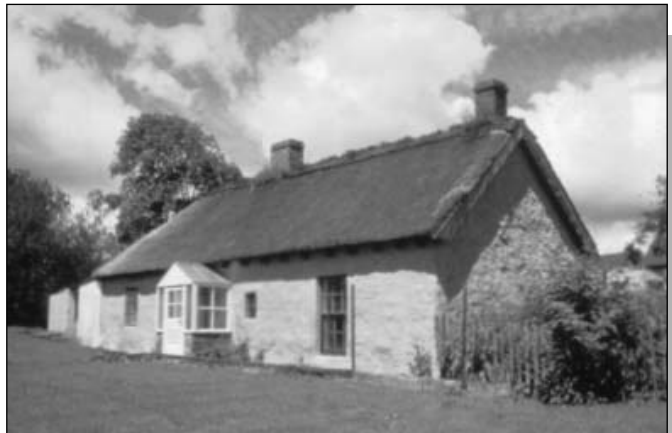
Figure 13.18: Recently renovated 200-year-old earth building in pisé construction in Perthshire. Source: Howard Liddell
