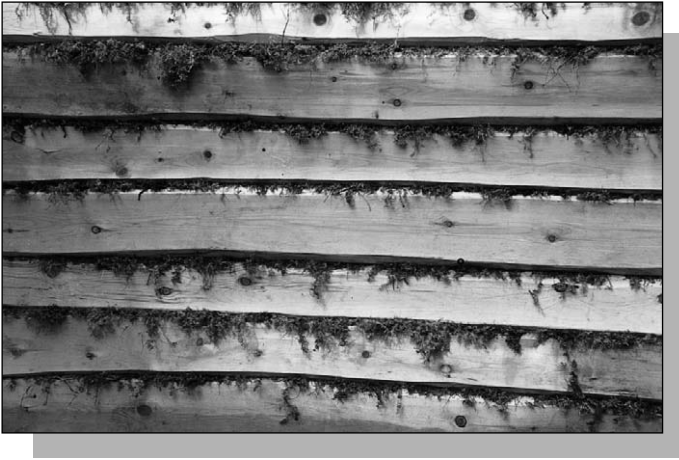
Figure 14.20: Log wall sealed with moss.
