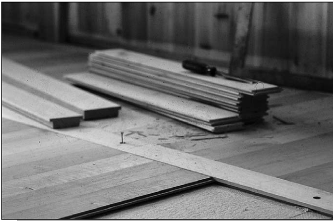
Figure 15.24: Batten flooring under construction.
