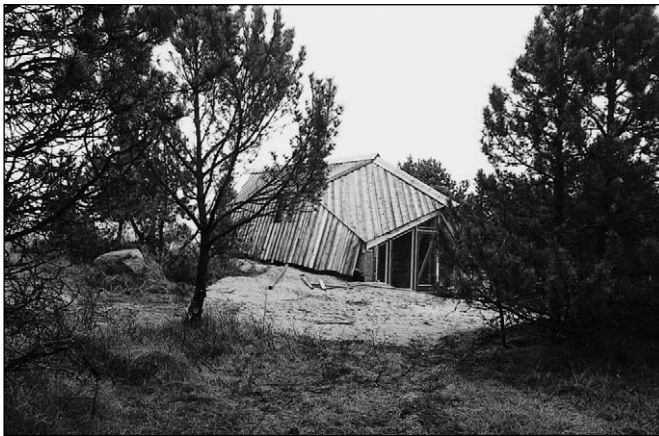
Figure 14.11: A cabin partly buried in a sensitive area along the south coast of Norway. The materials and structure have been chosen with respect to the climate, earth and water analyses. The aim has been to reduce the physical and chemical traces of the building to a minimum when it finally disappears. Source: Gaia Lista, 1997
