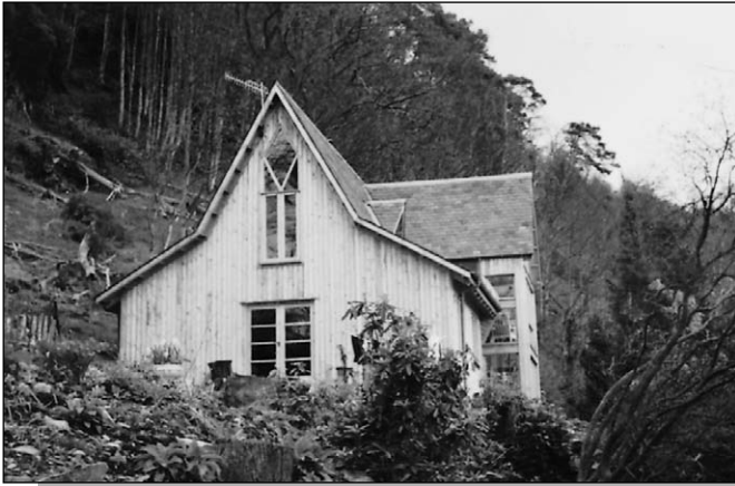
Figure 15.2: A house with a recycled slate roof in Aberfeldy, Scotland. Source: Gaia Scotland 1993
