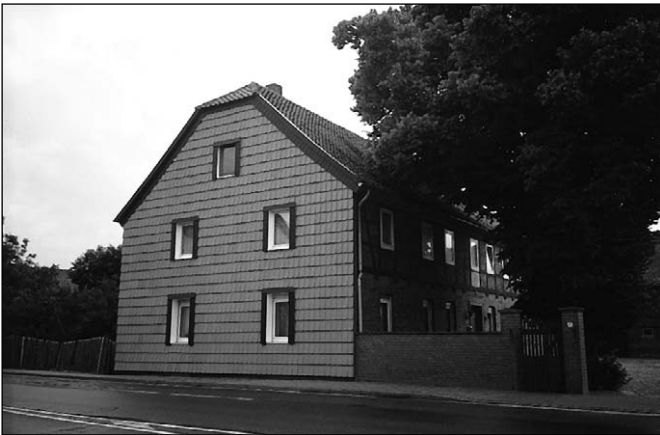
Figure 15.6: Facial cladding with clay tiles.
