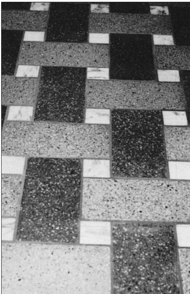
Figure 15.1: Floor of terrazzo slabs with marble tiles.
