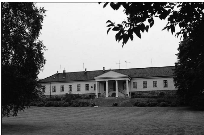
Figure 13.26: The manor house of Skinnarebøl in south east Norway from the early 19th century is built in the wet-formed wall technique.
