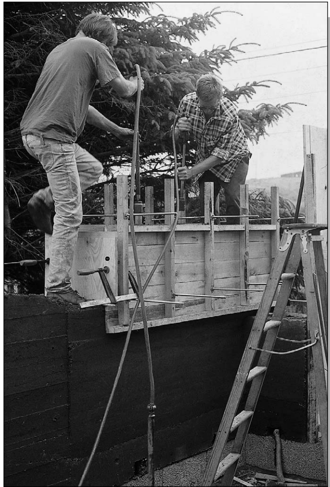
Figure 13.20: Ramming earth with a compressed air machine. Source: Gaia Lista 1991
