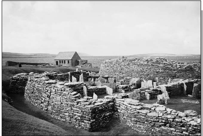
Figure 13.6: The remains of a traditional dry-walled structure in Ireland. Source: Dag Roalkoam
