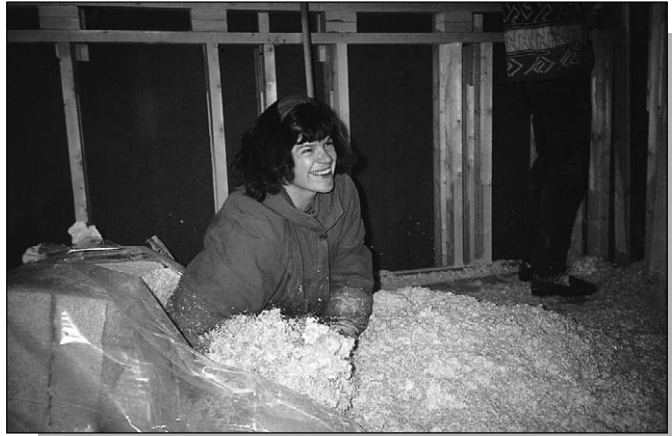
Figure 14.12: Thermal insulation made out of sawdust.
